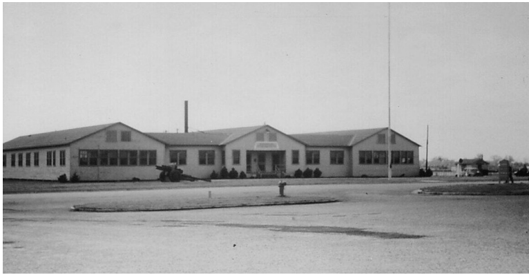
The Base Headquarters building located in front of the Base Chapel and behind Fire Station #1. Note the very tall 125' flag pole.
